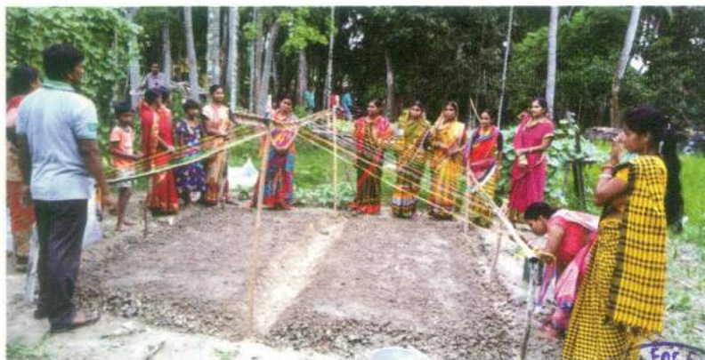
Handholding Training on Construction of Rainshelter
