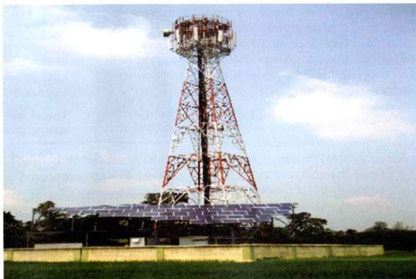
Hybrid power supply to telecom towers
